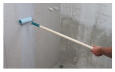
${f 1}$  The substrate must be clean, flat, dry and load bearing. Priming the substrate is recommended.
