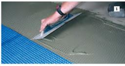
■ APPLY LOOSELY MIXED MODIFIED THINSET TO THE SUB-STRATE USING A 1/4" × 1/4" NOTCHED TROWEL.
