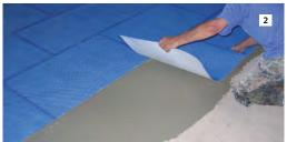
■ INSTALL BLANKE PERMAT FLEECE-SIDE DOWN, MAKING SURE TO OVERLAP AND KEEP 3" MIN. OFFSET PATTERN.\*
