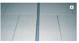
■ REMEMBER TO INSTALL PERIMETER JOINTS AND BLANKE EXPANSION JOINTS PER TCNA GUIDELINES EJ171.\*\*
