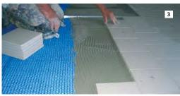
■ WORK THIN-SET MORTAR INTO THE SURFACE OF BLANKE PERMAT AND SET THE TILES.
